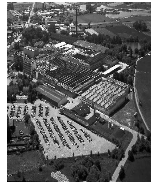
Stiebel Eltron plant in Holzminden, Germany
